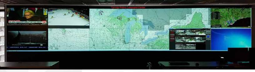
The primary purpose of a display wall in any control room is to provide Situational Awareness and a useful large Common Operating picture for multiple operators to simultaneously see relevant information (data, graphics and video) and collaborate in critical decision-making processes.
